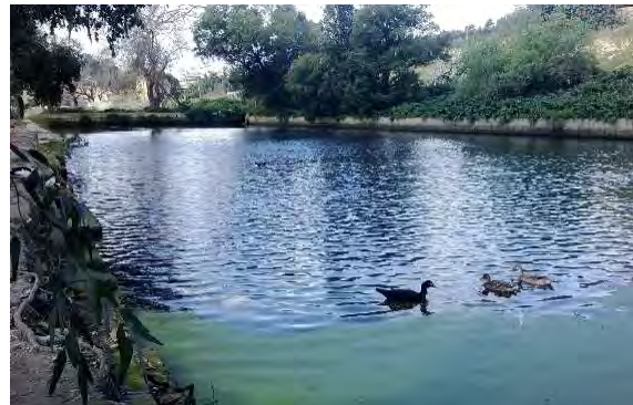
Figure 20: Soakaway at Msida
