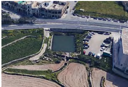
Figure 19: Soakaway at Żebbuġ
