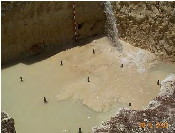
Figure 61: Borehole wells at MDH soakaway under test
