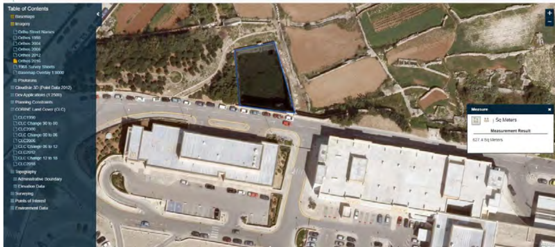
Figure 59: Aerial photo of the soakaway with a footprint of 400 m 2 at Mater Dei Hospital (MDH)
