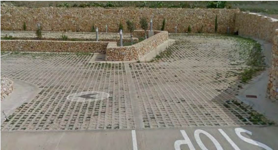
Figure 80: Permeable pavement at Għarb, Gozo
