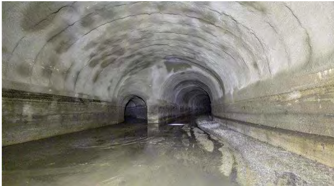
Figure 31: NFRP internal view of a tunnel confluence
