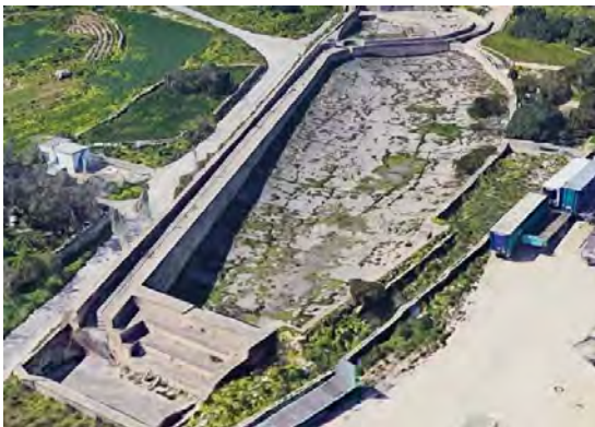
Figure 21: Soakaway at Ħas-Saptan
