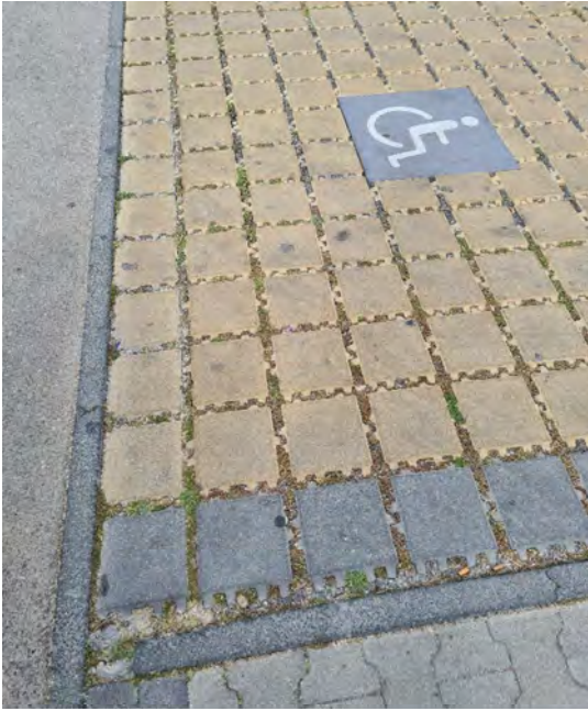
Figure 78: Permeable pavement at Mosta
