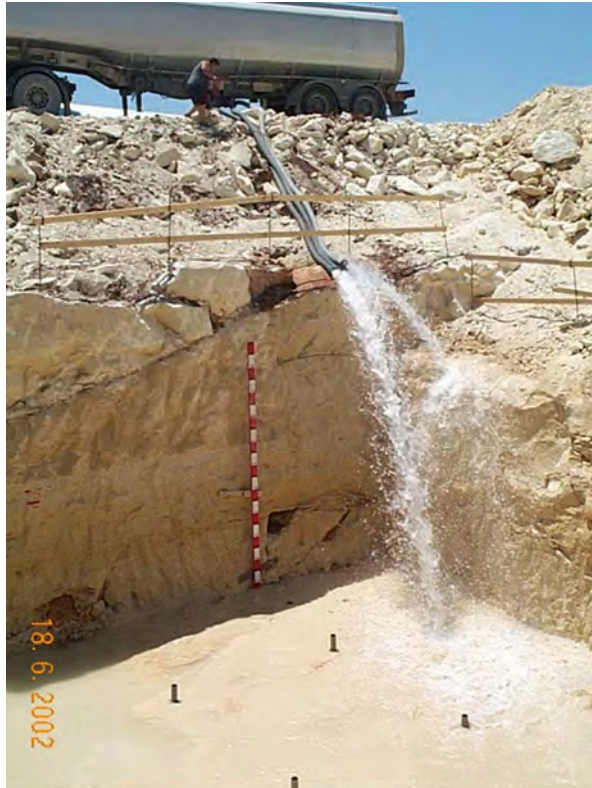
Figure 60: MDH soakaway under test
